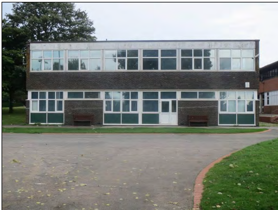
Plate 2.21 Extreme western end of the southern elevation. This block is situated at the lowest level of the western incline. This elevation optimises the use of external prefabricated wall panelling and continuous glass window panelling at both stories, facing north (6959-0051)
