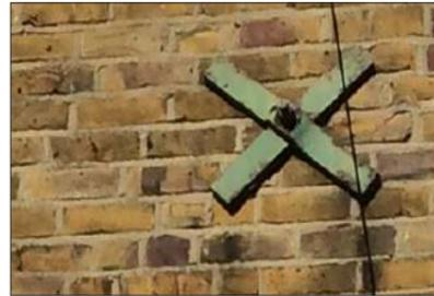
Existing Bracing Metal Detail
